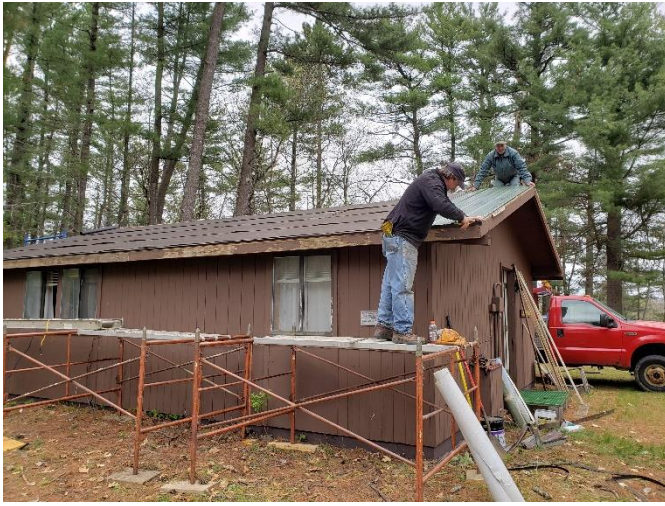
New roof added to Director's Cabin.
