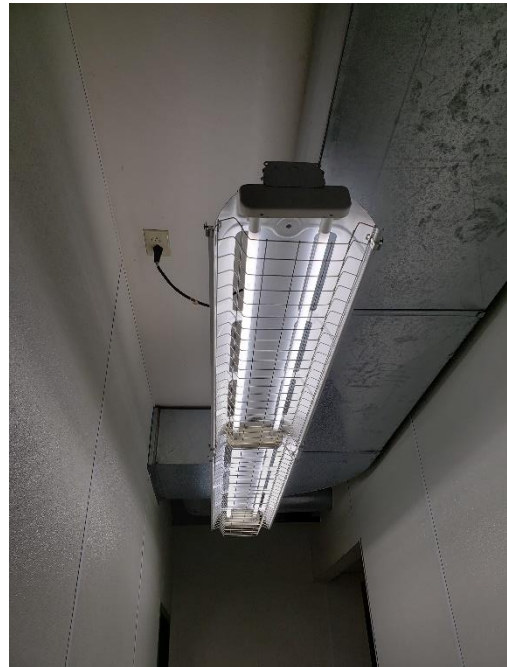
Lighting improvements completed in the kitchen of Dahl Dining Hall.
